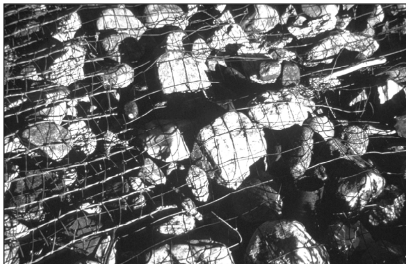
Figure 1.5. Wire-Enclosed Riprap
