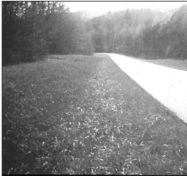
Figure 1.2. Vegetative Channel Lining
