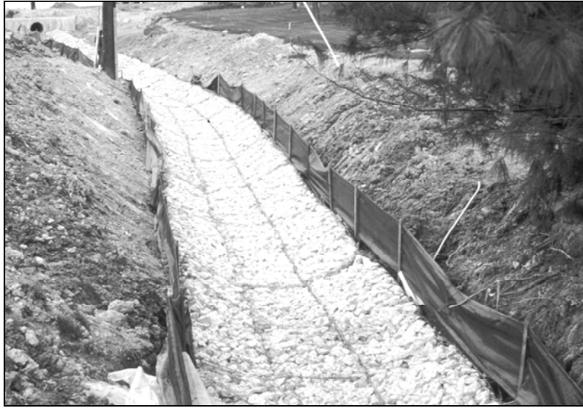
Figure 1.6. Installed Wire-Enclosed Riprap
