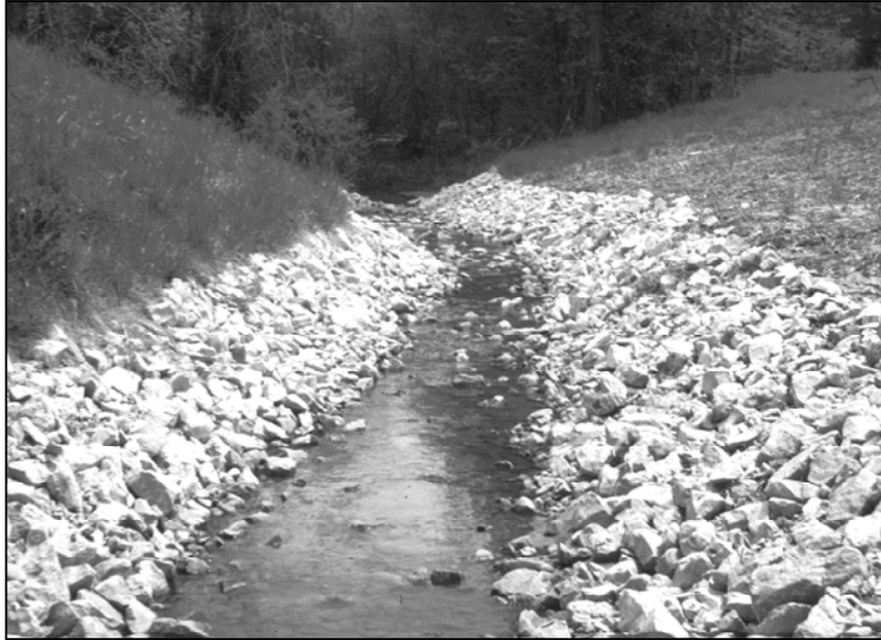
Figure 1.4. Riprap Channel Lining
