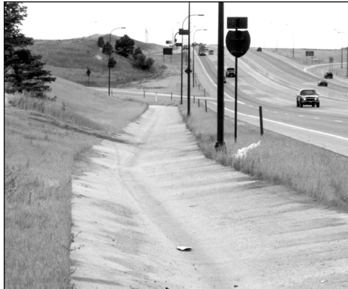
Figure 1.1. Rigid Concrete Channel Lining
